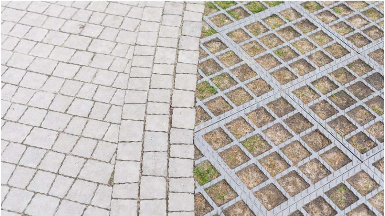
Figure i. Two examples of permeable pavements. Photo credit: U. S. Environmental Protection Agency.
