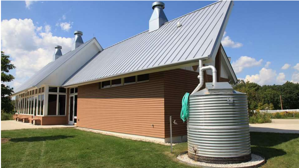
Figure b. A cistern connected to a rainwater collection apparatus and roof. Photo credit: U. S. Environmental Protection Agency
