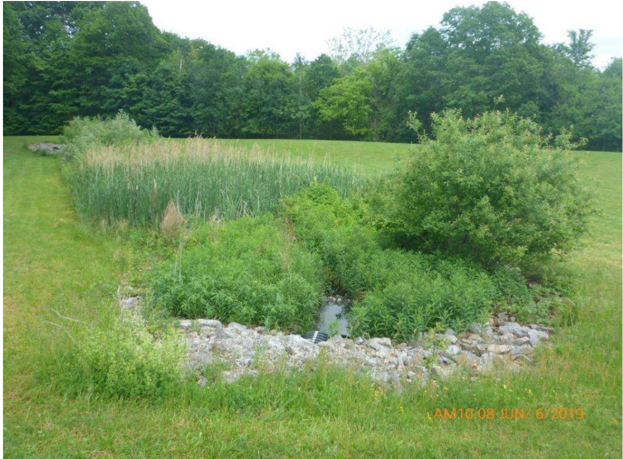
Figure k. A vegetated filter strip can infiltrate and treat stormwater flow from adjacent surfaces using a variety of plants. Photo Credit: Steven Chase for U. S. Environmental Protection Agency, 2019.
