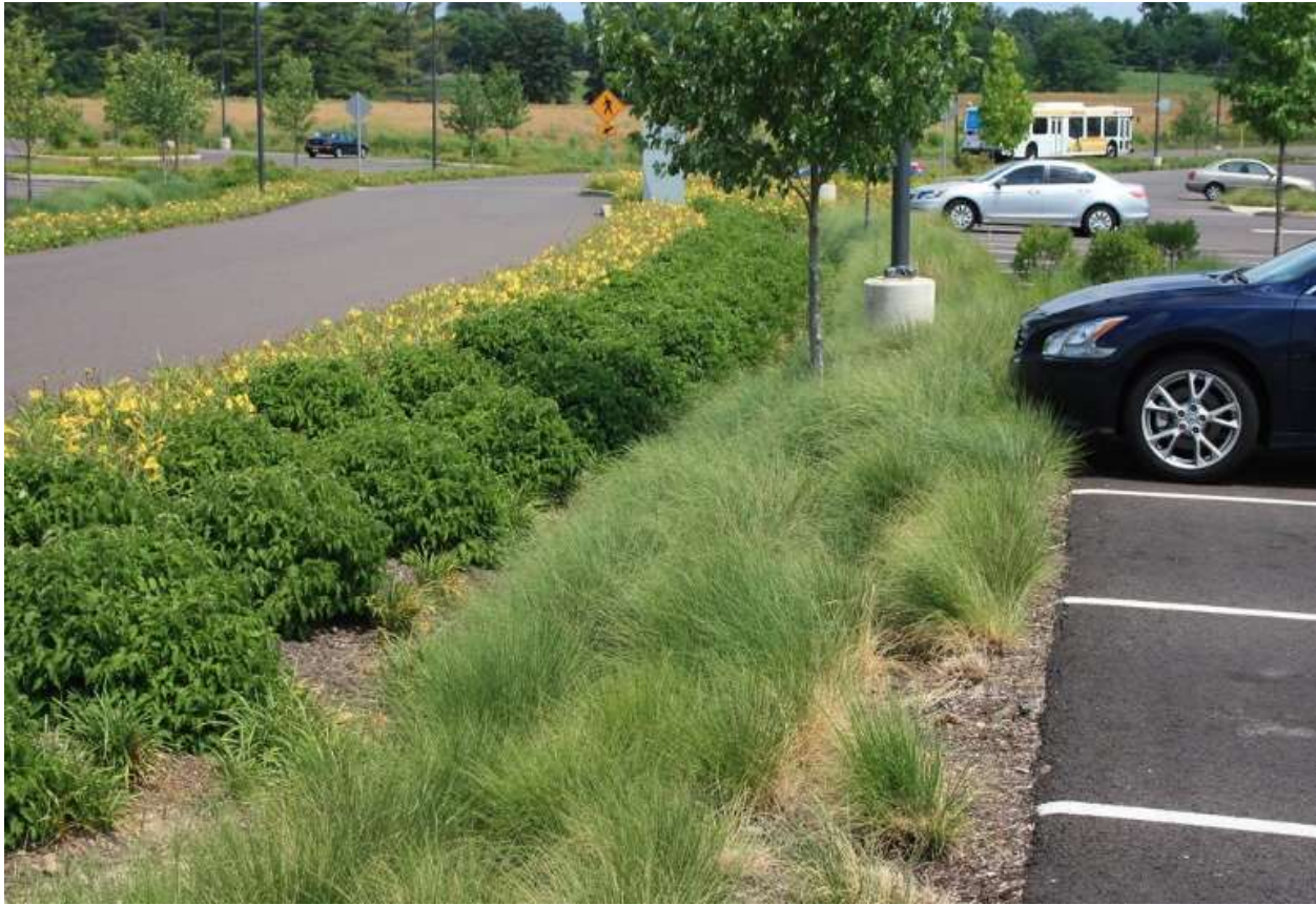
Figure h. Infiltration trenches at Einstein Hospital in East Norriton, Pennsylvania. Photo credit: U. S. Environmental Protection Agency.
