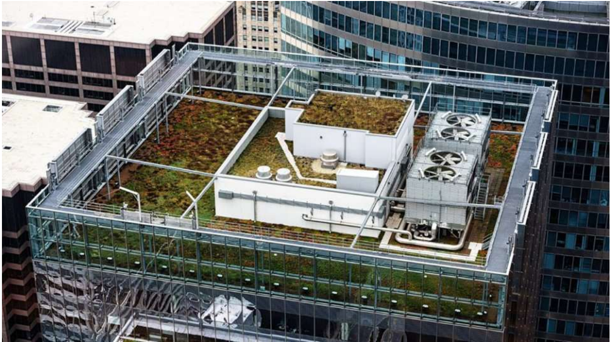
Figure f. An urban building with planted segments on its rooftop. Photo Credit: U. S. Environmental Protection Agency.
