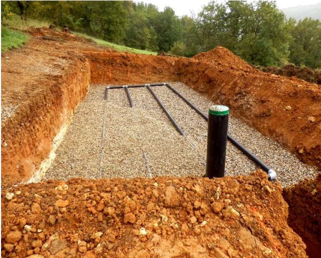
Figure j. A sand filter under construction. Photo credit: U. S. Environmental Protection Agency.
