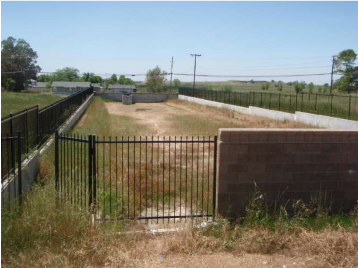
Figure d. A dry detention pond with security fencing. Photo Credit: U. S. Environmental Protection Agency.
