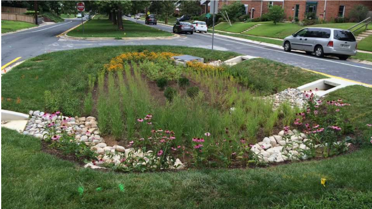
Figure a. A bioretention practice in a suburban road median. Photo credit: U. S. Environmental Protection Agency
