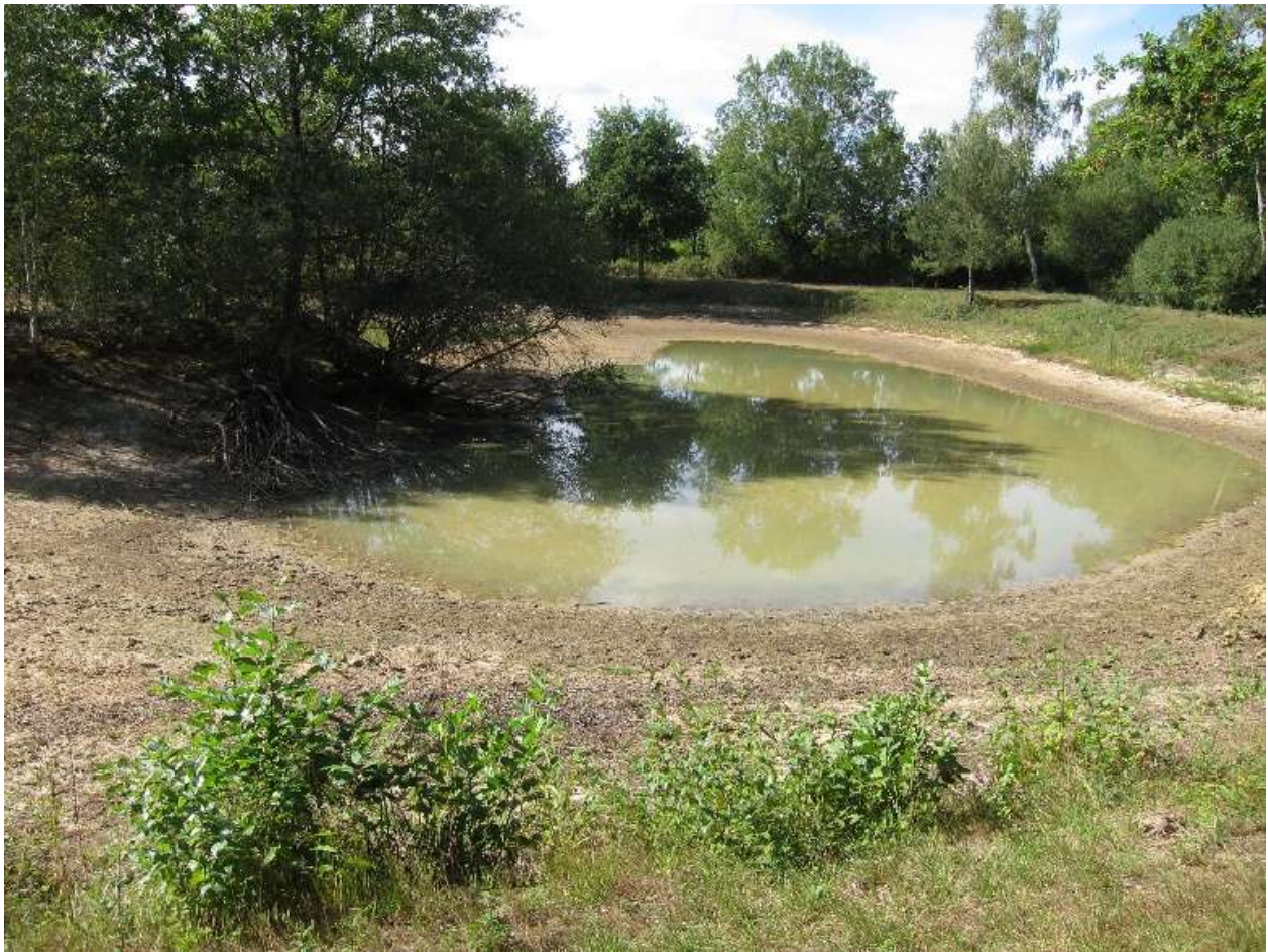
Figure g. Infiltration pond in a natural area. The infiltration portion consists of sand with a high infiltration rate. Photo credit: U. S. Environmental Protection Agency.
